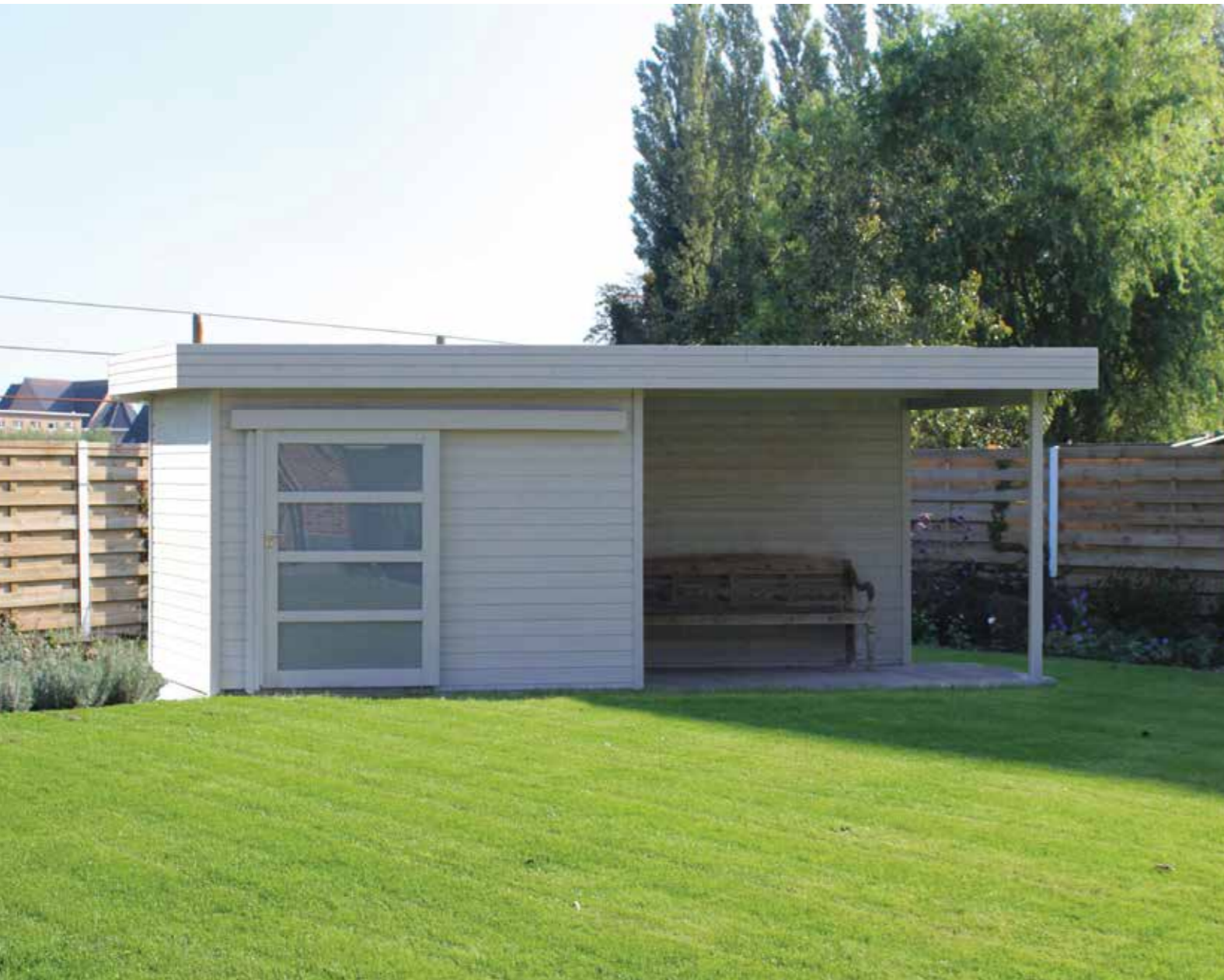
Modern in paneelbouw
